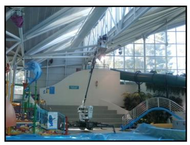
Given the length of time since the initial paint and the high humidity environment, significant corrosion was present to the Aquatic Centre steelwork. ProjectPlus's preparation needed to be thorough and precise prior to the application of the epoxy coatings
